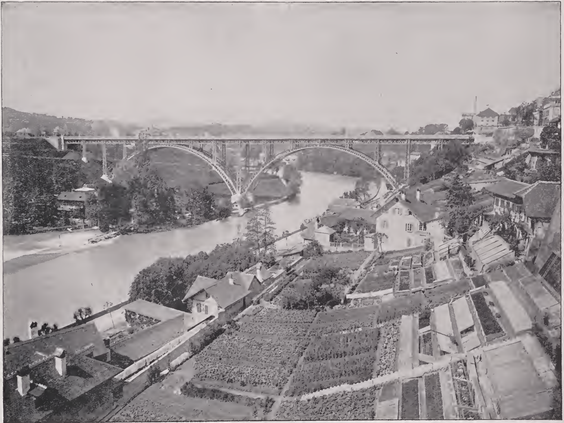
KIRCHENFELD BRIDGE, BERNE, SWITZERLAND.—The above structure is a huge iron bridge, seven hundred and fifty-one feet long, built in 1882-1883, across the river Aare, from the town proper to Helvetia Platz, where a new quarter of the town is being built by an English company. In the foreground are the terrace-like hot-houses and gardens of the peasants, who earn their livelihood by supplying the inhabitants of Berne with vegetables from their little farms. From the top of the bridge, in clear weather, the Bernese Alps can be seen better than from any other point in the Oberland.
